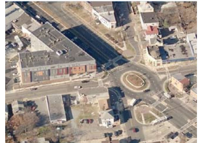
New mixed use infill and a roundabout along Rhode Island Avenue in Mount Rainier, MD
