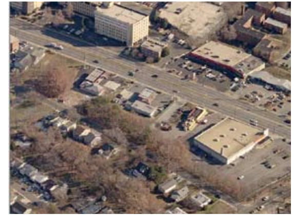
Existing birds-eye aerial view of the Maryland Gateway area with Sligo Mill Road in the foreground.
