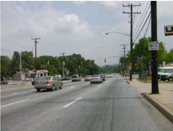
View looking north on New Hampshire Avenue towards MD 410 Intersection.
