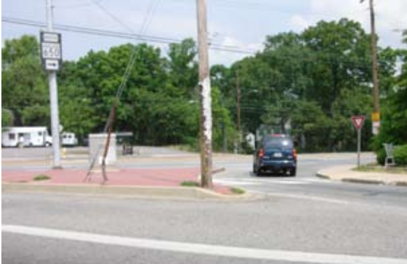
Intersections in the corridor have been designed for unimpeded vehicular flow.
