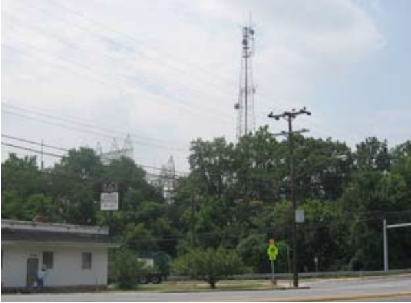
Looking southeast from New Hampshire Avenue towards the Animal Hospital and the PEPCO substation beyond.
